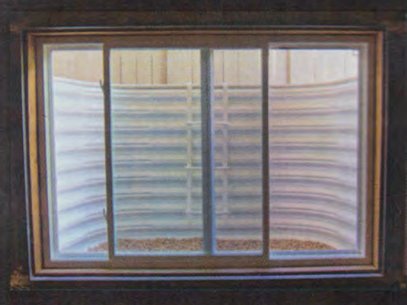
STEEL This galvanized material comes in one preformed piece, up to 60 inches high, which cuts down on installation costs. Many manufacturers offer built-in rungs for climbing out.
