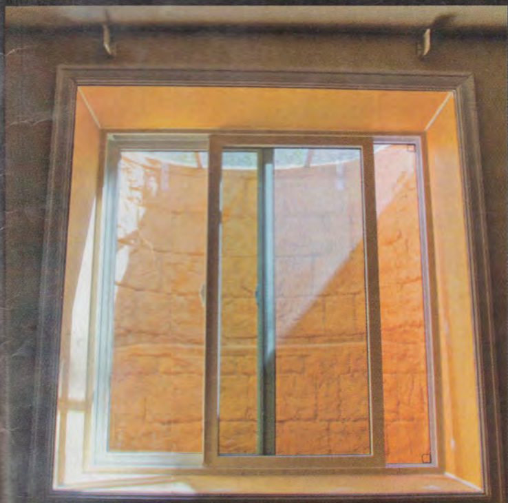
MASONRY Window wells made of concrete block, natural stone or precast concrete are the strongest and most durable option—best for cold-weather areas where soil heaving is common.
