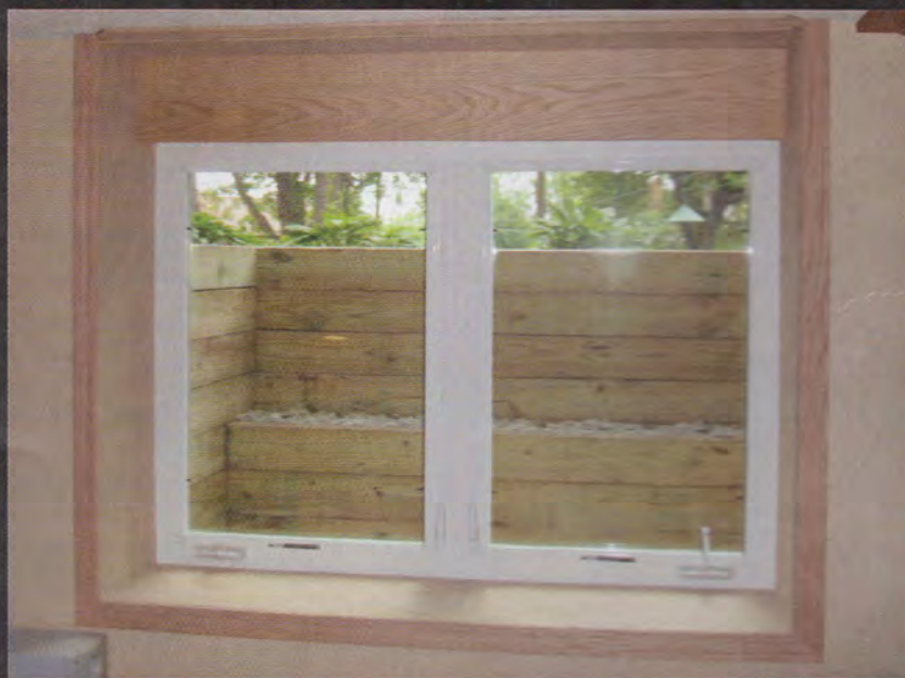
TIMBER FRAMED This traditional frame (covered by a see-through plastic shield) is a homeowner favorite, but it's important the installer use pressure-treated wood to avoid rotting.
